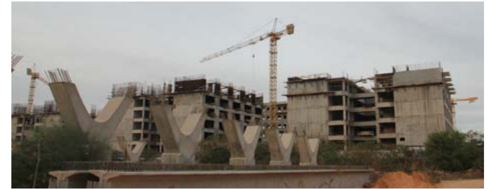
□ Tripoli unfinished motorway construction
