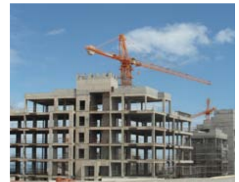
□ Building under construction, Tripoli
